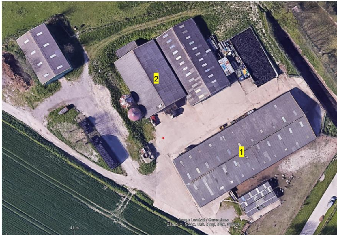
Figure 37: Google earth image of Ovingdean farm building roofs, labelled for solar potential analysis
