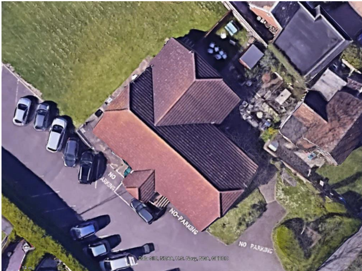
Figure 38: Google earth image of Ovingdean Village Hall
