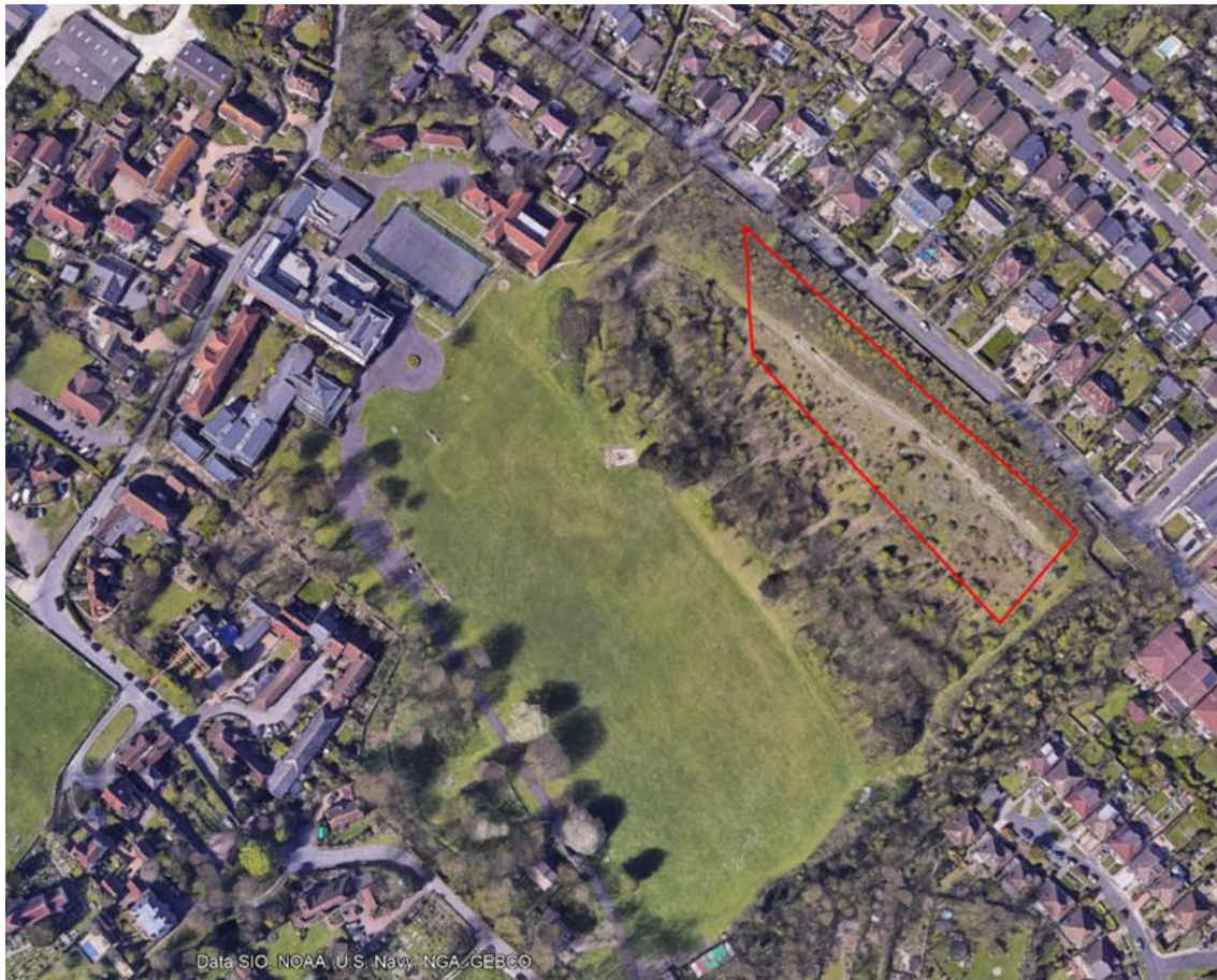
Figure 35: Land owned by Oxford International College that could be suitable for ground mounted solar as it's not used as playing fields
