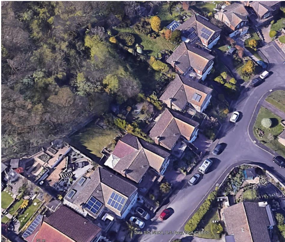
Figure 30: Google Earth image of Wanderdown Way in Ovingdean, where some homes have solar panels in different layouts
