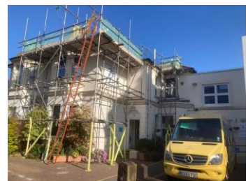
Solar PV install
